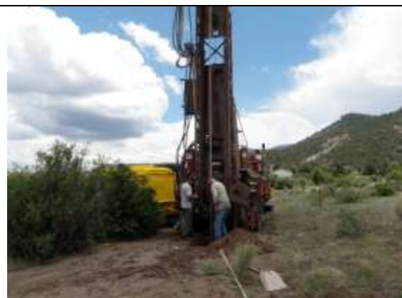
Setting pump on 1" pipe
