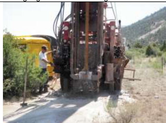
Drilling – groundwater blowing out of hole
