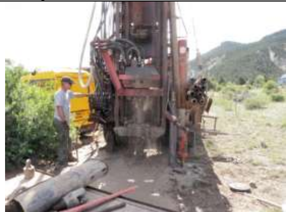
Drilling – groundwater blowing out of hole
