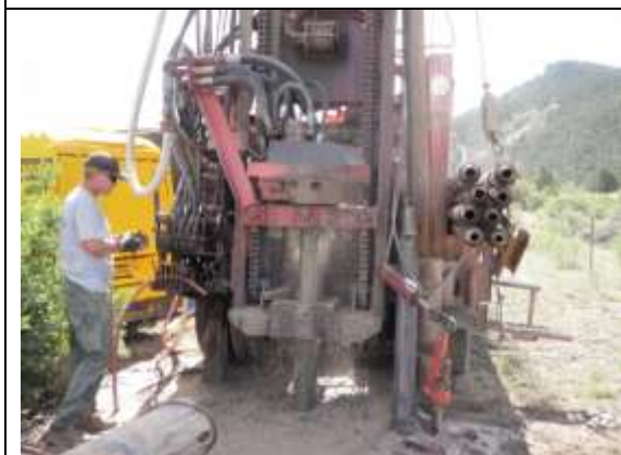
7/7/15 Hole is cased with 6 inch steel pipe
