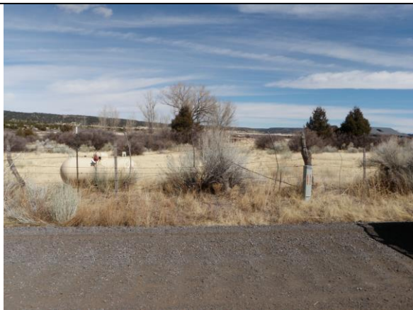
15. LPG tank and phone with fiber optic cable on CR
