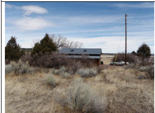
16. House, South side
