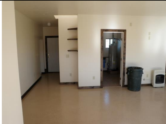
3. Bathroom, hall to bedroom & back door
