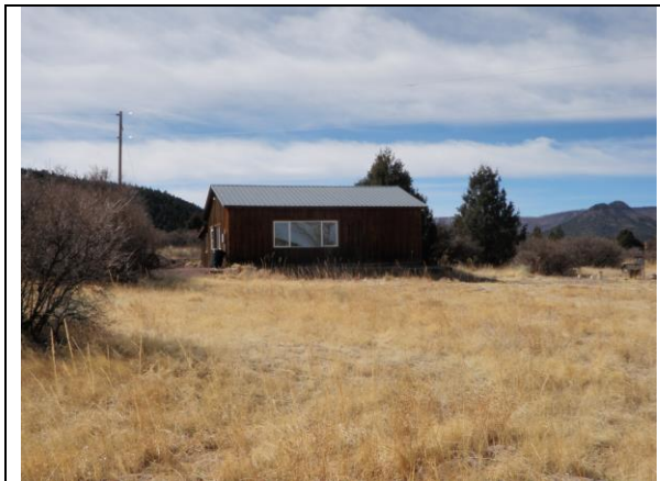
14. North side of house looking south
