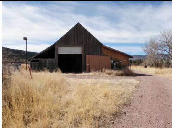
4. Barn, north side, 14 ft high x 12 ft wide roll up door
