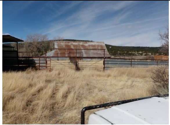
4. Barn and corrals from east side
