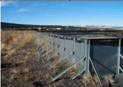
13. 250,000 gallon water storage tank
