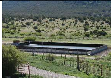
14. 80'x80'x4.5' water storage tank
