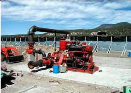
11. 380 HP Cummings diesel motor and pump
